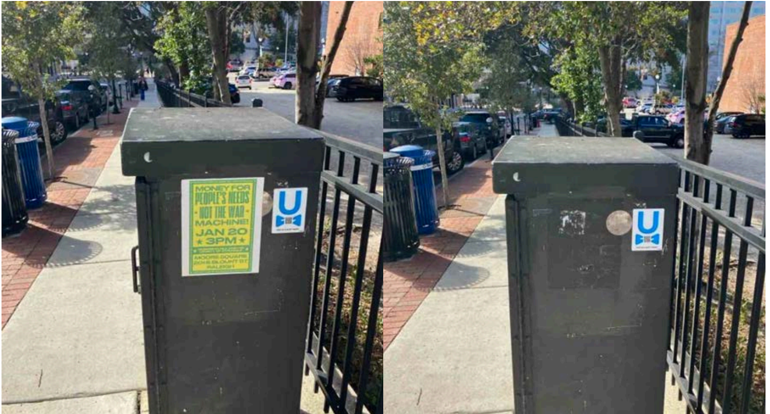
HANDBILL REMOVAL - GRACE STREET
