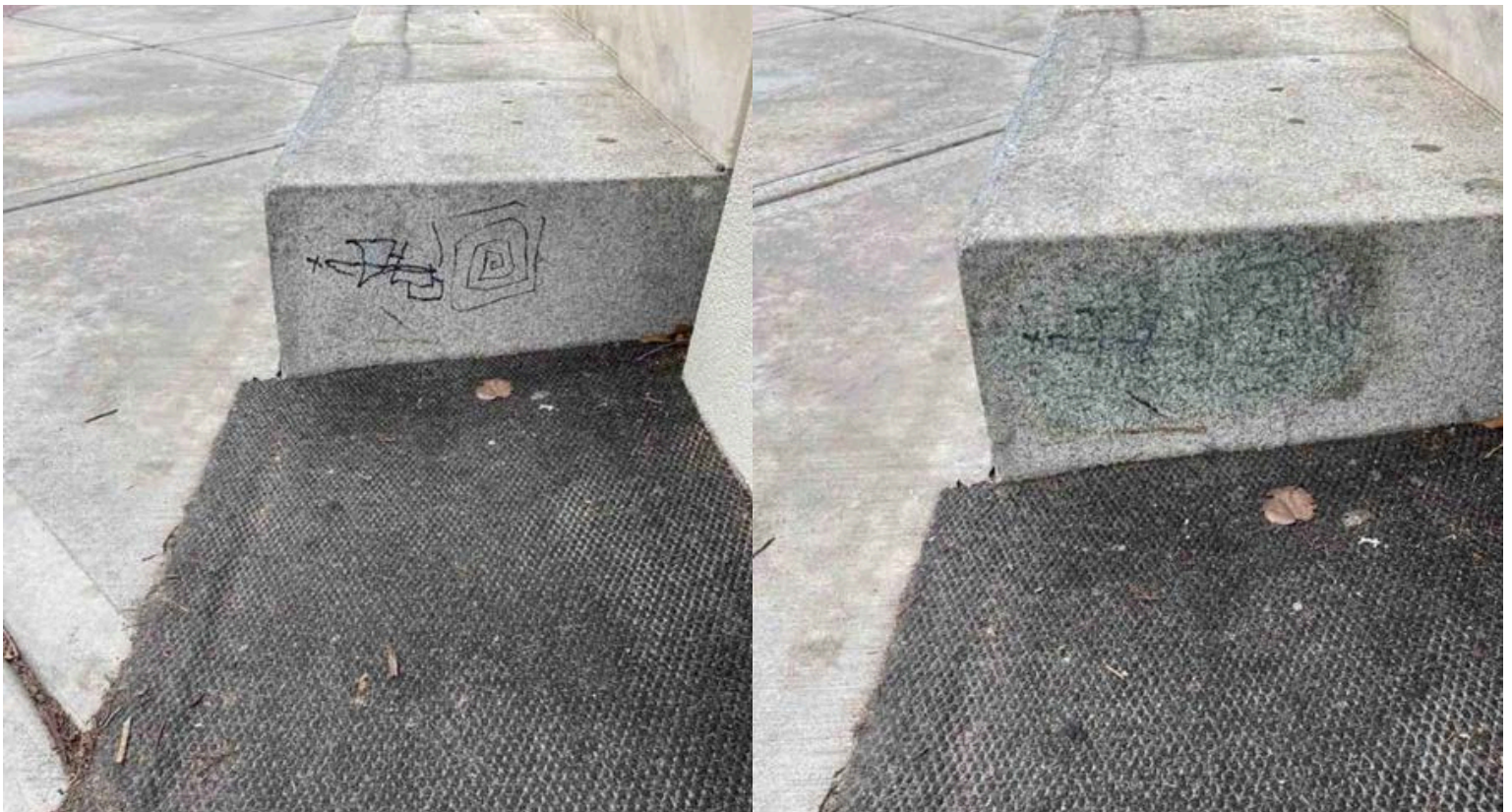
GRAFFITI REMOVAL – WATER STREET
