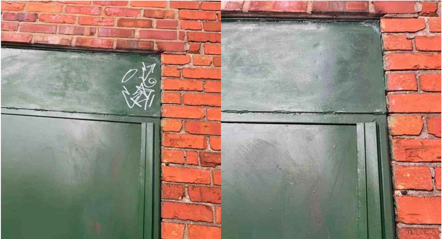
GRAFFITI REMOVAL – MUTTERS ALLEY
