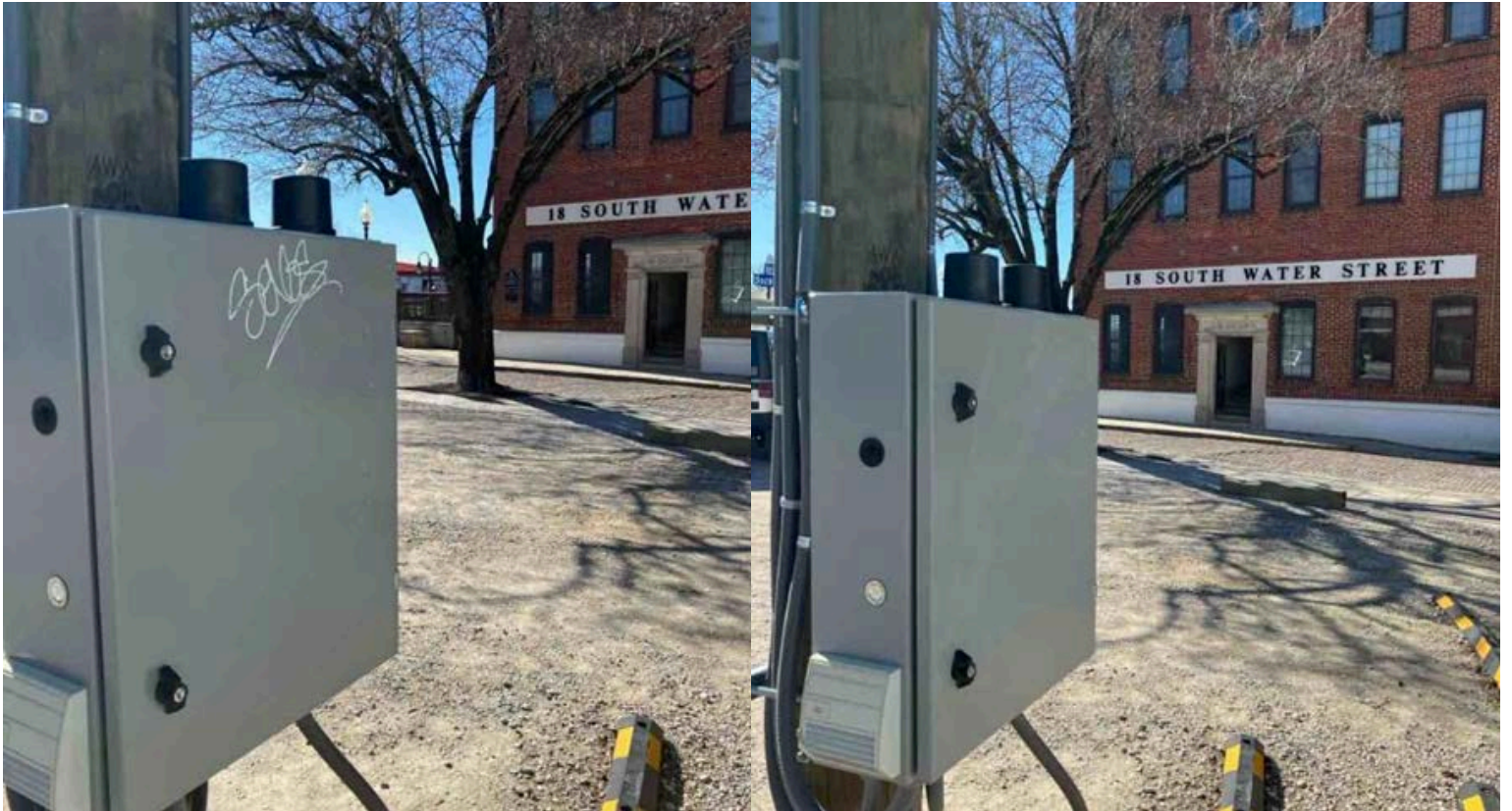
GRAFITTI REMOVAL – SOUTH WATER STREET
