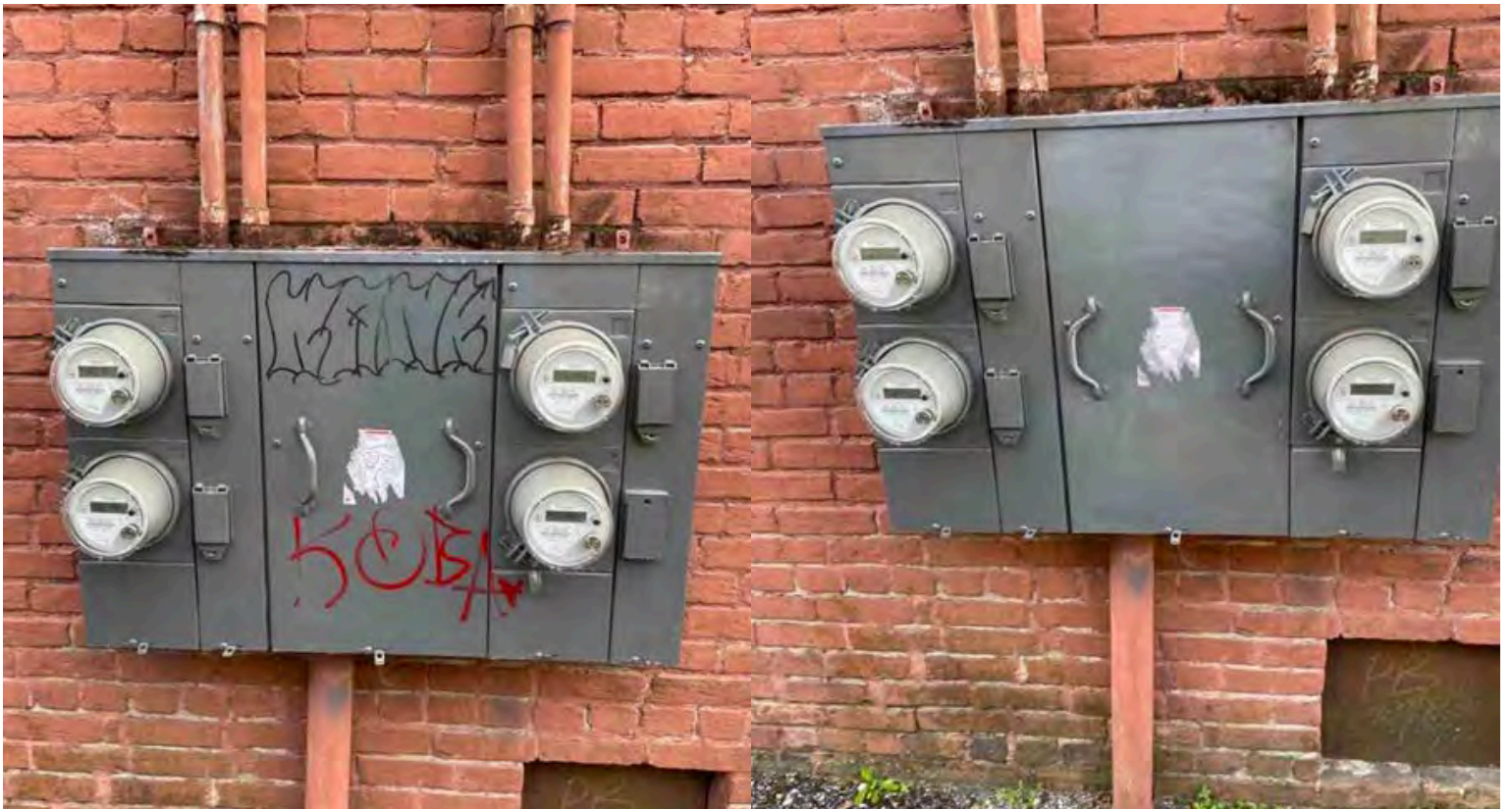
GRAFFITI REMOVAL – VANCE ALLEY
