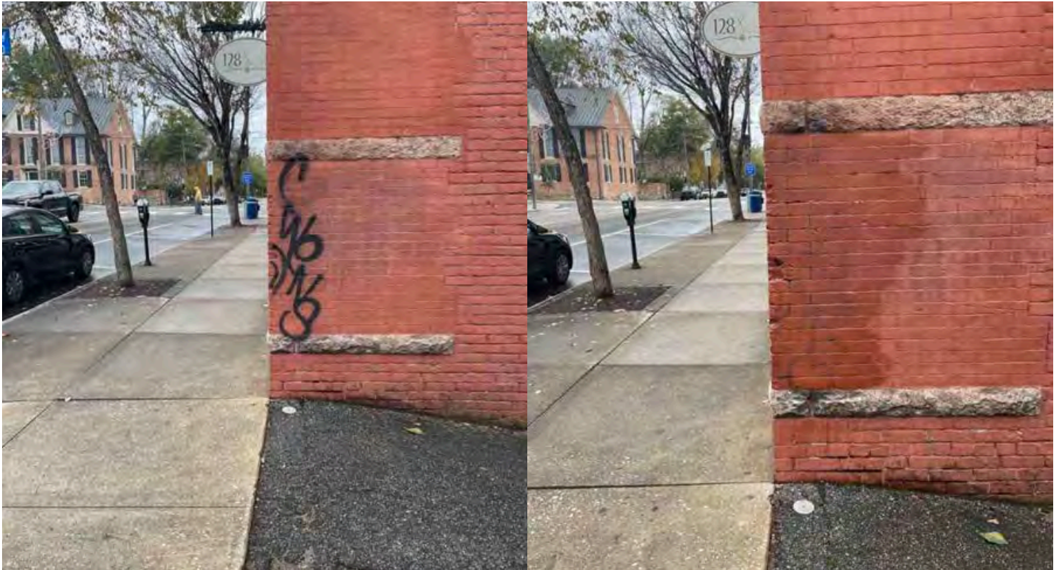
GRAFFITI REMOVAL - FRONT ST
