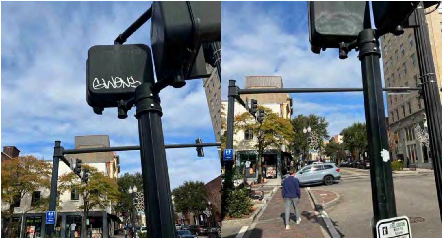
GRAFFITI REMOVAL – FRONT ST
