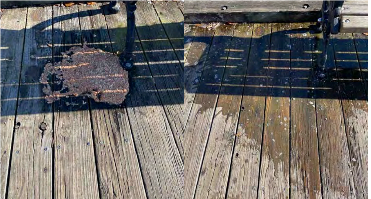
BIOHAZARD REMOVAL – RIVERWALK
